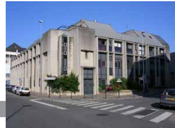
France Telecom - Daubenton
