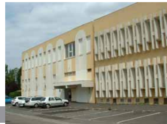
France Telecom - Merignac
